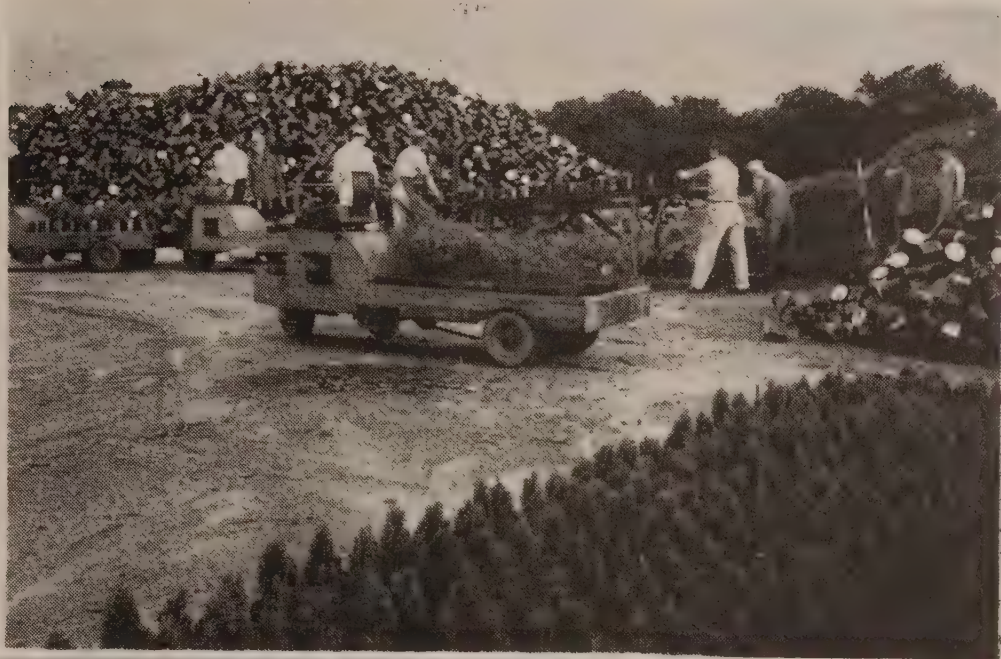
Our new efficient "Canning Machine" for planting 1-gallon can stock.
